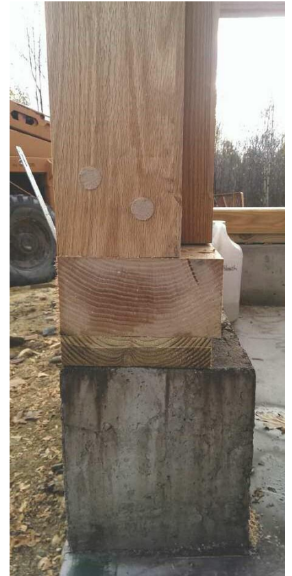
Post on sill on frost wall.
