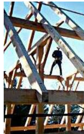
Rafters are installed.
