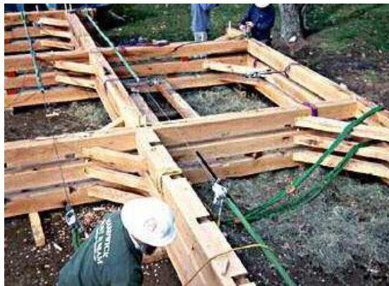
Bents ready to be raised.
