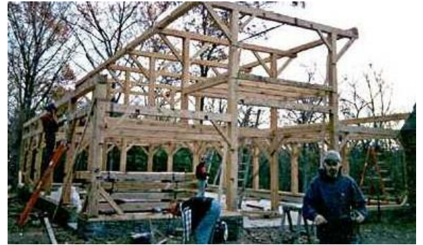
Plates are connected to the bents.
